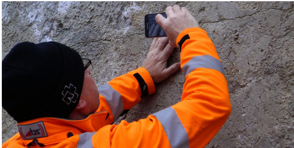
Crack inspection. © J. Denis
